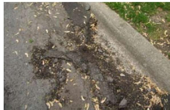
As you know, the curbs are in poor condition and crumbling in many places. Moreover, the repeated application of slurry seal over the original surface means that they are now very low relative to the grade of the street in some areas, creating drainage problems. There's no way to mill down the street surface and repave without destroying
